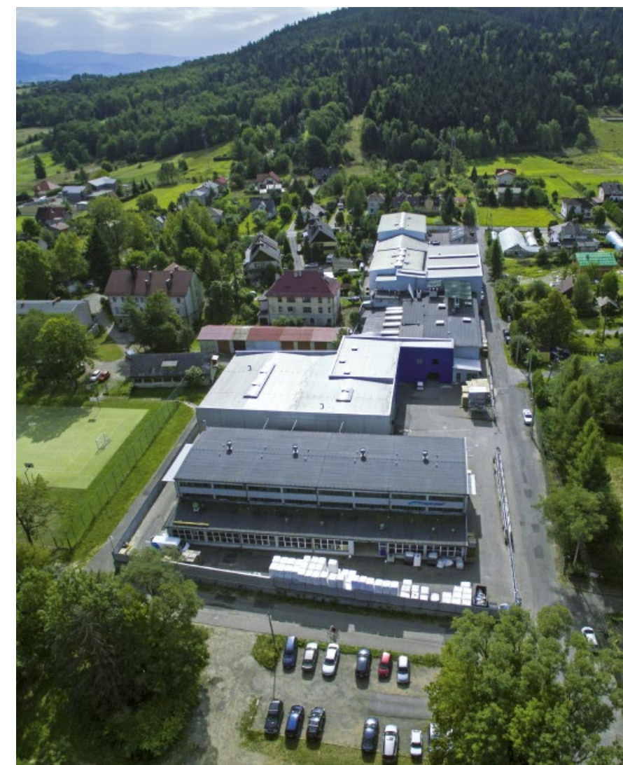
Buczkowice – production & warehouse
