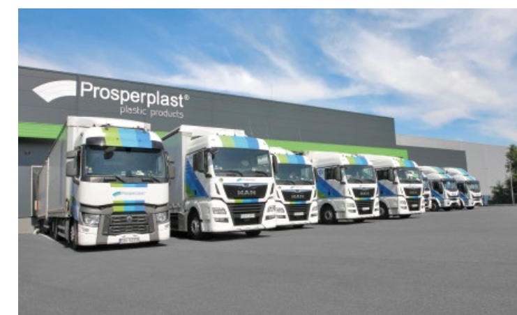
Wilkowice – logistic centre
